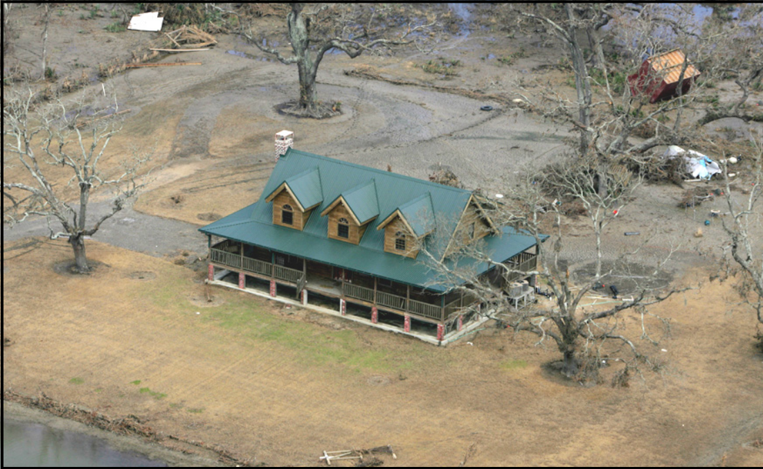
Sheila and Clayton Mhire's home in Grand Chenier, La., built with blueprints and logs from Heritage Log Homes of Sevierville, withstood 120 mph winds and a 15-foot storm surge during Hurricane Rita.
